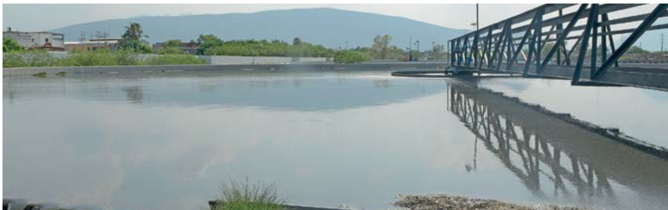
The "Northern" wastewater treatment plant in Monterrey, Nuevo León. May, 2016.
