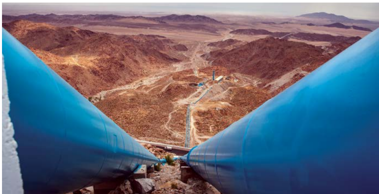
The Río Colorado aqueduct in Tijuana, B.C., with a view of pumping plants 5, 4 and 3.
