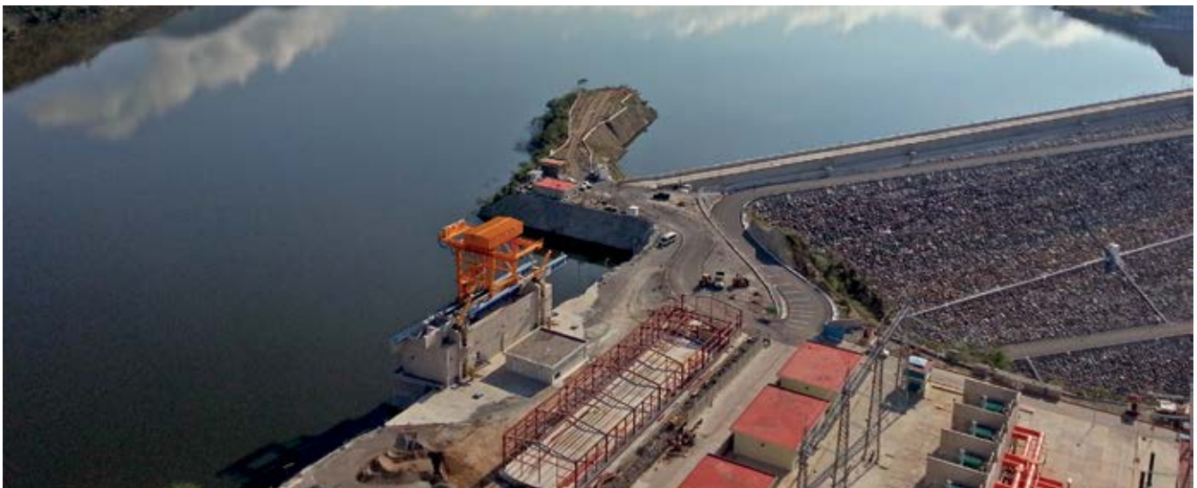
Aerial view of the "La Yesca" dam, located in the Río Grande de Santiago, in the municipality of La Yesca, Nayarit, and Hostotpaquillo, Jalisco
