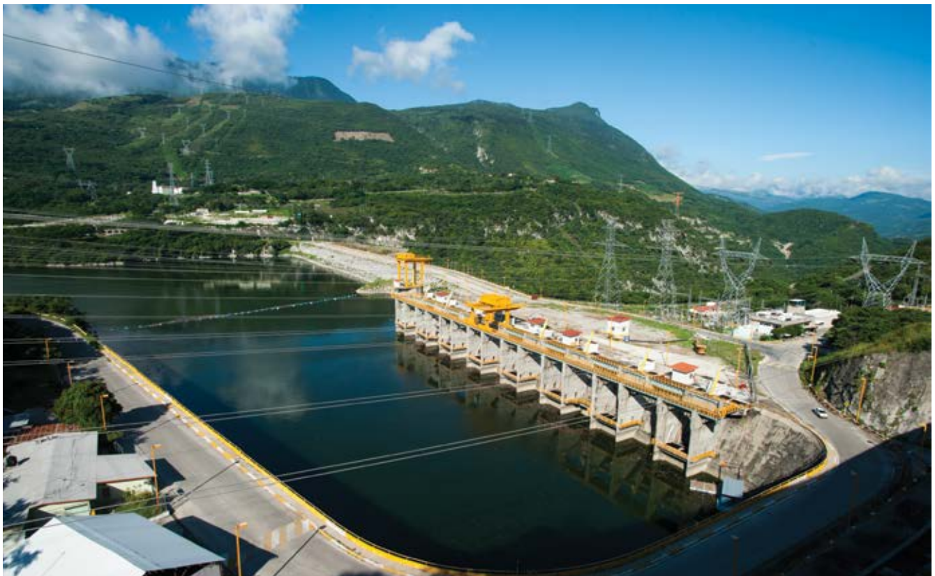
The Manuel Moreno Torres "Chicoasén" hydropower plant, Chiapas, part of the Grijalva River hydropower system.
