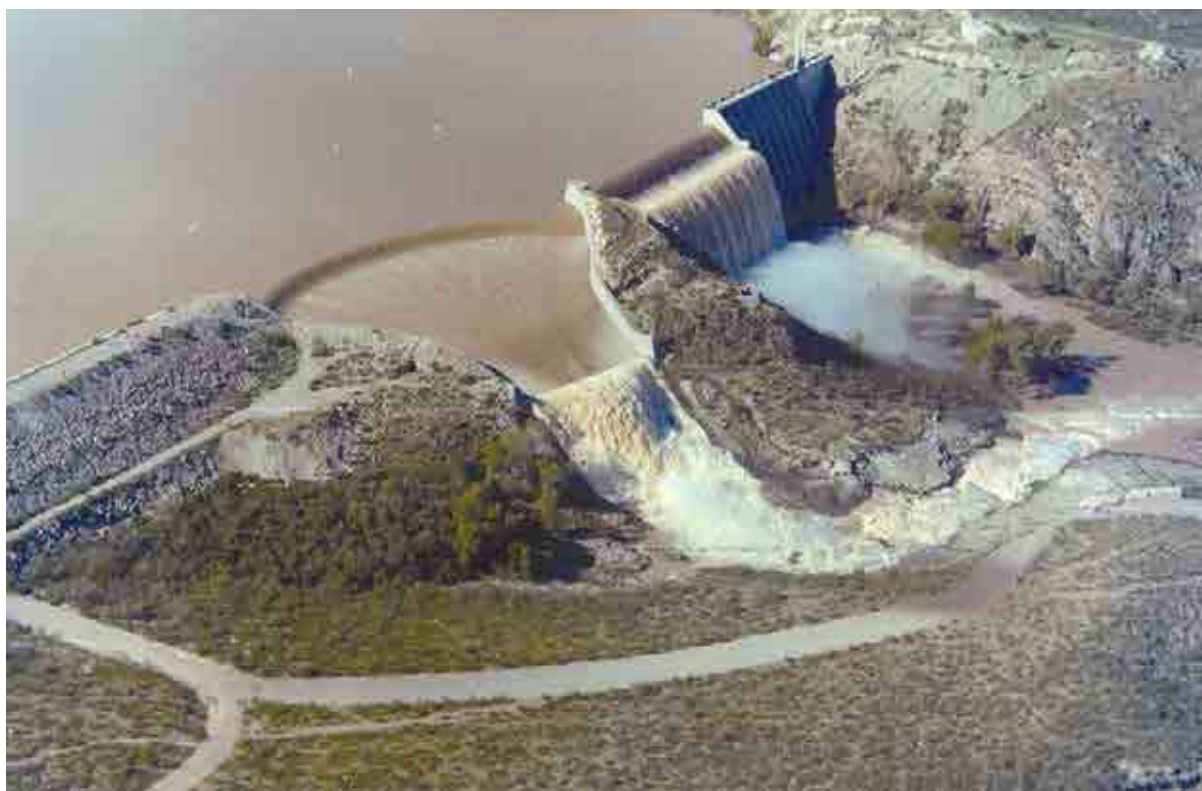
Photograph of the Francisco I. Madero dam, also known as Las Virgenes, Municipality of Rosales, Chihuahua, 1949
